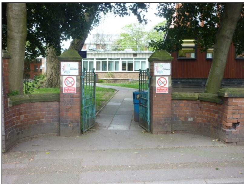
P11 - Base of T37 & T38 abut existing boundary wall causing displacement. Trees appear dark & oppressive - removal will open up the area & allow for some new landscape enhancement works
