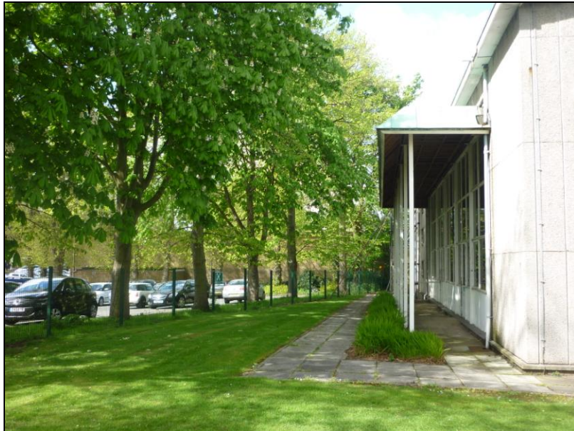
P9 - T24-T30 viewed from within the site. Canopies to be pruned back where necessary to provide a minimum 2m easement to new building
